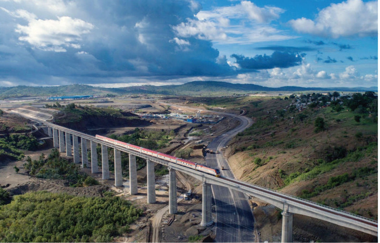
Aerial view of the Madaraka Express at Mazeras Bridge of the Mombasa-Nairobi standard gauge railway in Kenya (Photo Credit: Xinhua Photo)
