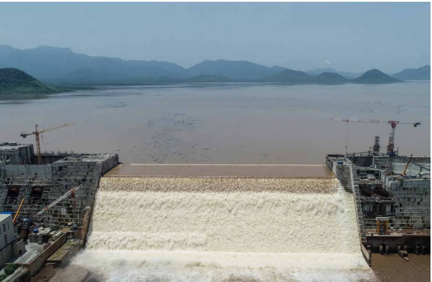
Aerial view of Grand Ethiopian Renaissance Dam on the Blue Nile River in Guba as of February 15, 2021 (Photo Credits: Adwa Pictures/AFP)
